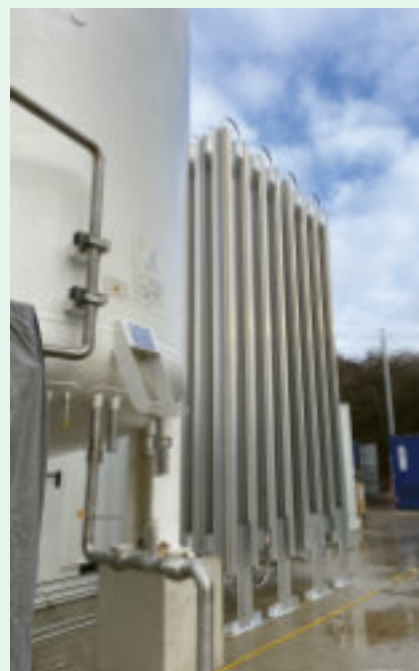
The air to air vapouriser
