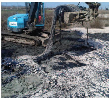
over to a vibrating shaker to further filter out stones and small items of vegetation. From there it was pumped over to a two phase centrifuge to separate the liquids and solids. The centrate was collected in a centrate tank where it was sampled for oil quality, water and solids contents; then pumped into six hundred tonne holding tanks where the oil and water separated over 48 hours.
